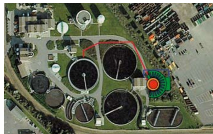
The wwtp of Terneuzen, including the projected upgrading with an airlift MBR
