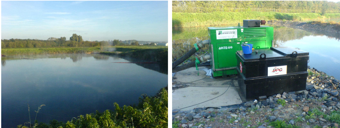
Figure 2. Impression of stabilization pond and pump to transport buffered effluent to the UF-RO plant.
