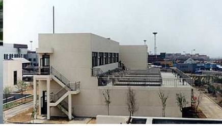
再生水厂滤池WRP Filtration
