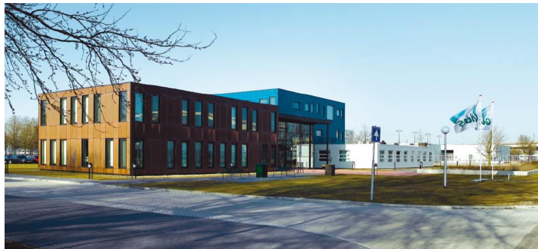
Headquarter of Evides in Rotterdam
